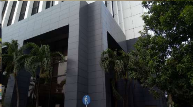
Gedung Kementerian Perindustrian, Jakarta Selatan (Revitalisasi ACP, Glass Cleaning Services)
