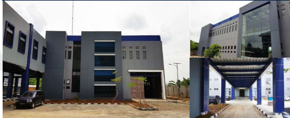
Kantor / Gudang Bea & Cukai, Cikarang (ACP, Aluminium Windows, Curtain Walls)
