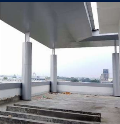
JIEP Financial Centre, Pulogadung (Curtain Walls, ACP)
